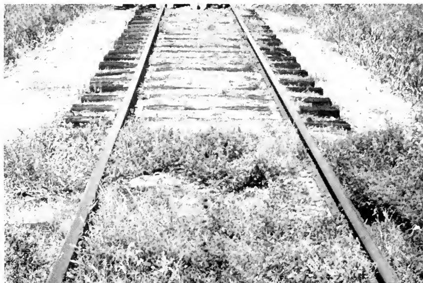
Fig. 2—Control of resistant roadbed vegetation in Florida with four applications of TCA, 40 lb-chlorate, 80 lb. It should be possible to keep this track clear with 2 treatments a year after the first year.
